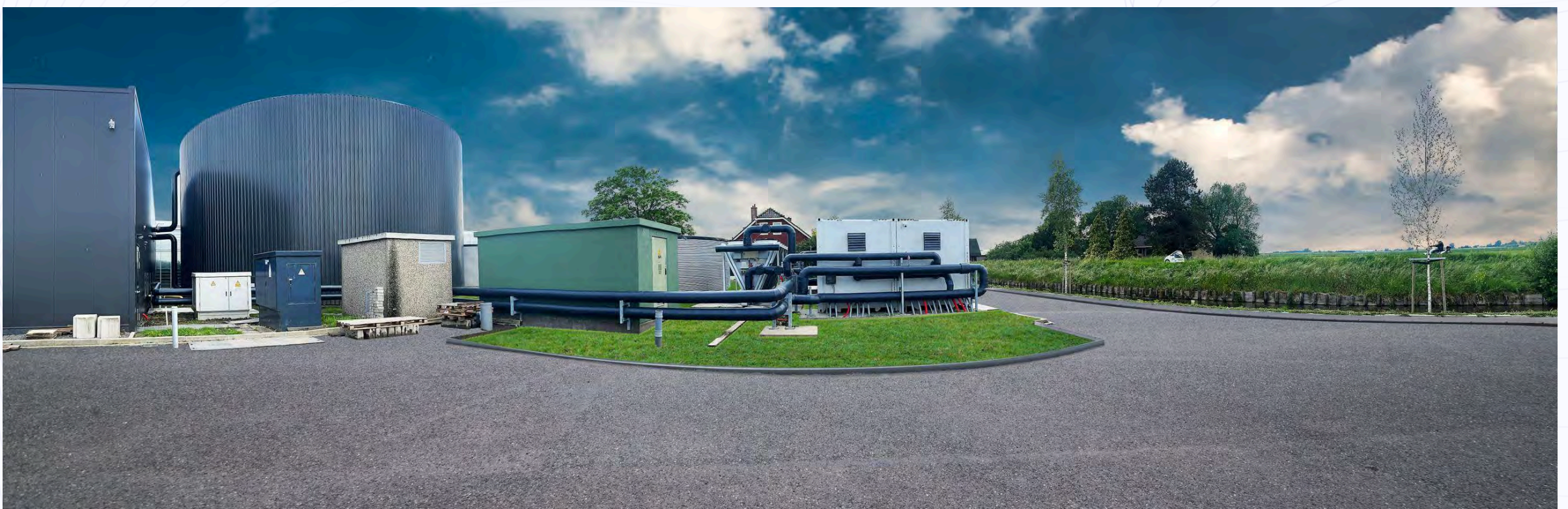
Sustainable heating solutions for growers (Source: GreenTech.Technologies)
